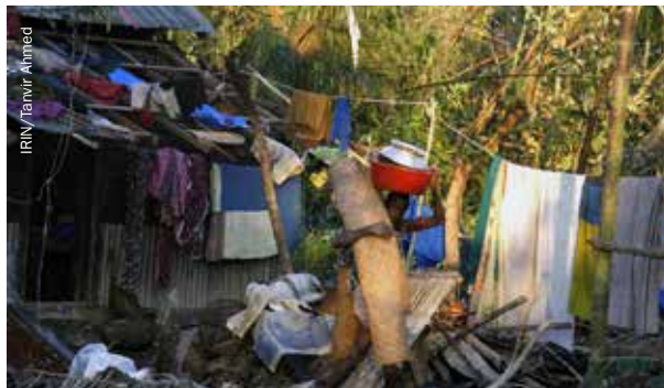
A cyclone-devastated home in southern Bangladesh, 2007.
